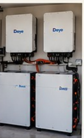
06 | BUNAWAN, AGUSAN DEL SUR 12kW Dual-Inverter + 30kWh
