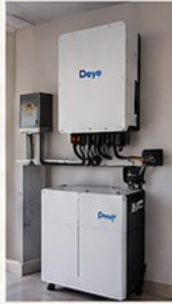
01 | UPPER CARMEN, CDO CITY 6kW Hybrid + 16kWh LiFePO4
